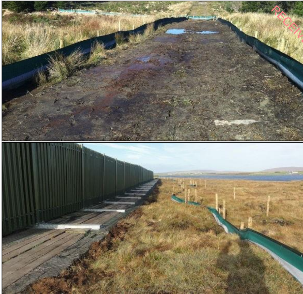
Plate 4: Typical Silt Fence Details
