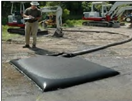
Plate 1 Silt bag under inspection
