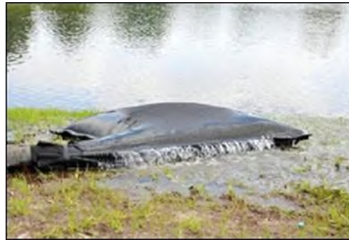
Plate 2 Silt bag with water being pumped through
